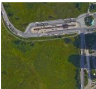
Hurdman Construction site – Before audit
